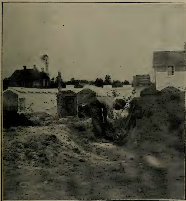
5.— Mixing soil. Breaking and pulverizing the sod preparatory to putting it down with layers of manure.
